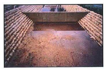
Multi-chamber structure consisting of a pretreatment chamber, a sand bed as Description:
