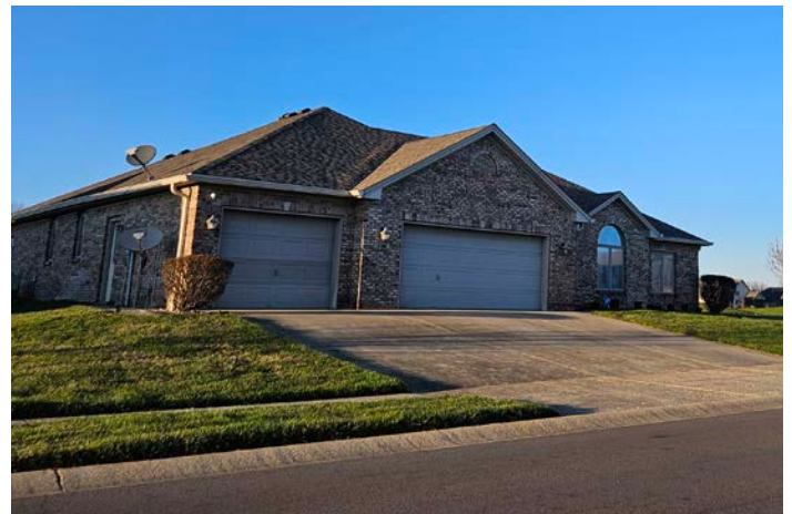
A home in the Timbergate subdivision. Image Source: HWC Engineering
